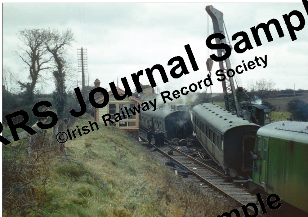
Figure 11. At a later stage of the lifting operation shown opposite, the damaged coach has been swung away from the Up line towards the siding, immediately opposite the wholly undamaged signal cabin. The locomotive is A42. (Photo © NJ McAdams - IRRS Collection)
