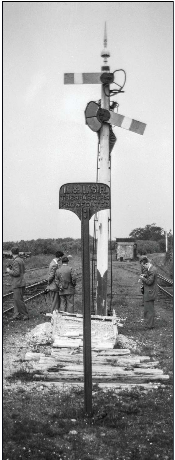
(above) The junction signal at Tooban Junction in June 1953, beyond which the separate branches of the L&LSR diverge to Letterkenny (left) and Buncrana (right). Note the heavy L&LSR trespass notice. (Photo © George Mahon - IRRS Collection)
