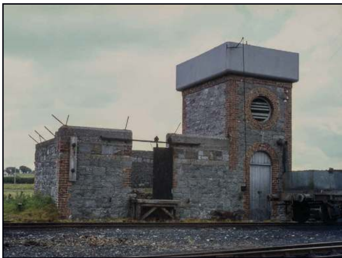
The disused stone built water tank (capacity 6,106 gallons) and coal staithe at Loughrea, photographed on Wednesday 14 August 1968. These structures were almost identical to those found on the MGWR's sister branch line to Ballinrobe. (Photo © Norman Gamble)
